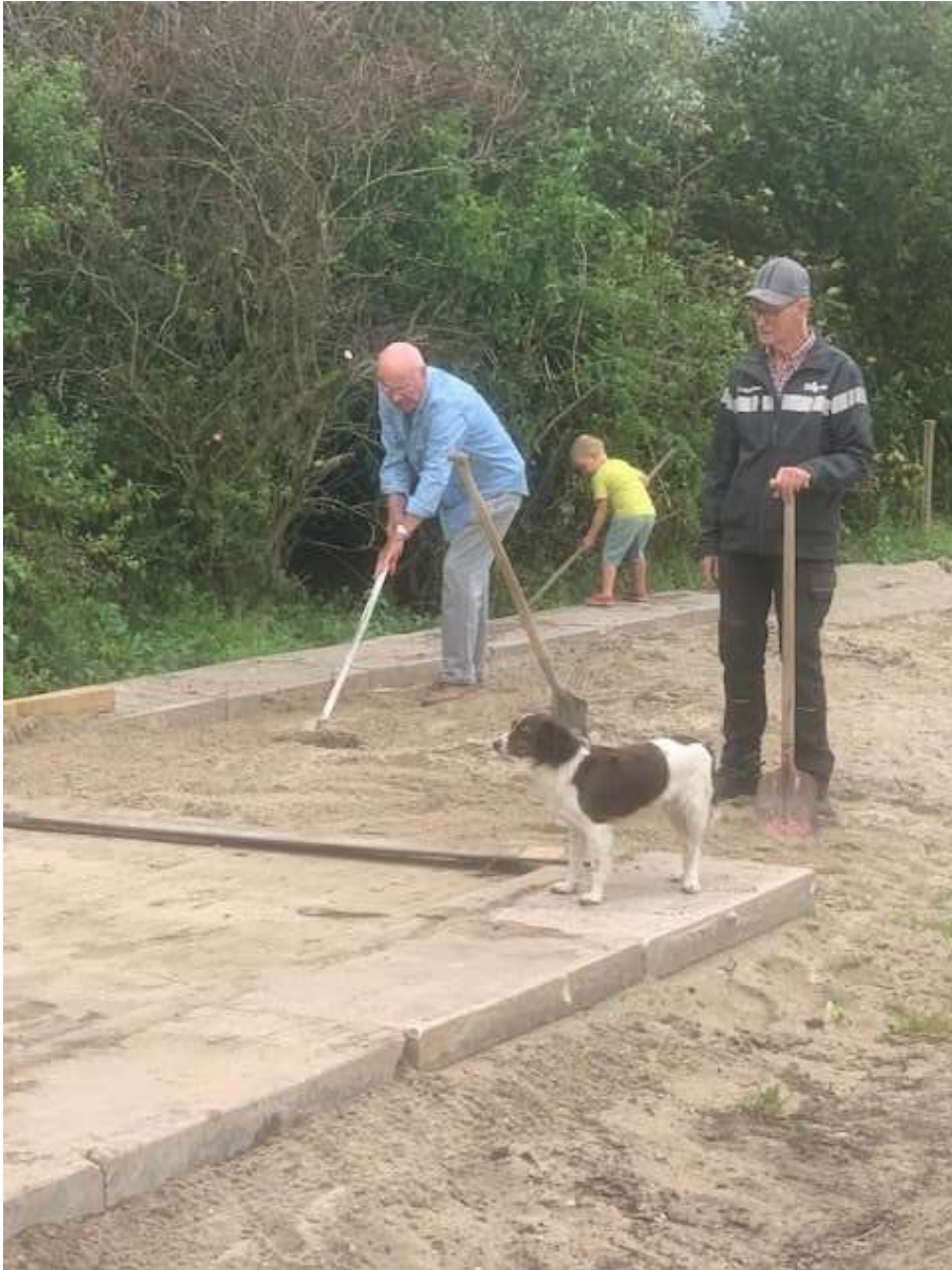
Project kippenhok is nog in volle gang.
